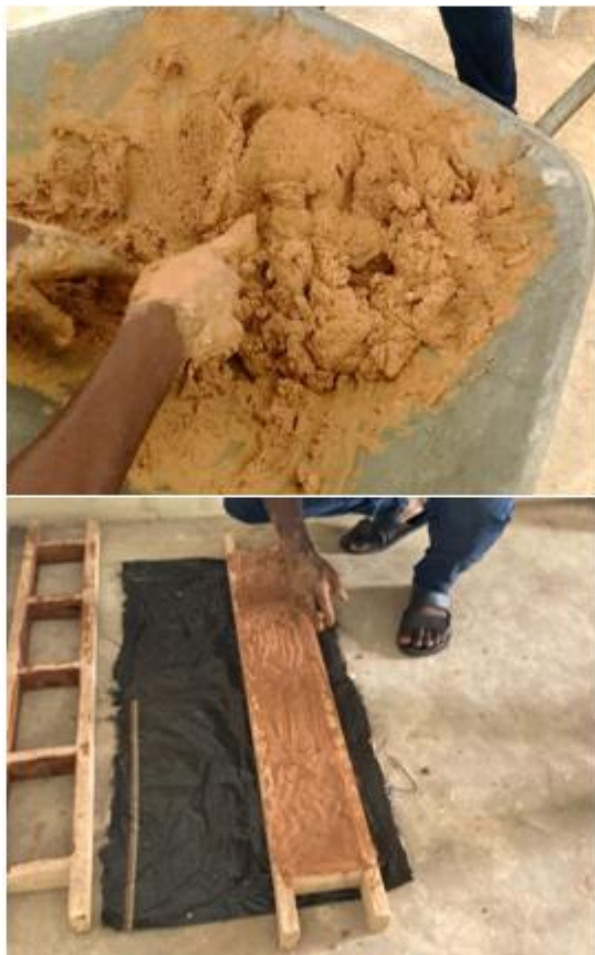
Figure 4: Mixing and casting the bricks
